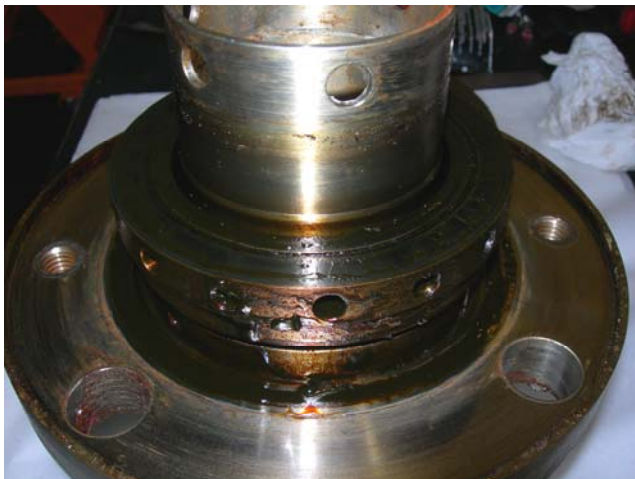
Fig. 3 Outboard rotary seal ring in-situ showing heavy oil tar build up.
